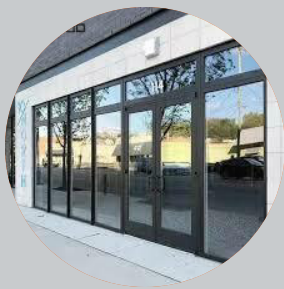
EXTERIOR LOADED ENTRY
