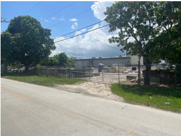
View of Subject Facing Southwest
