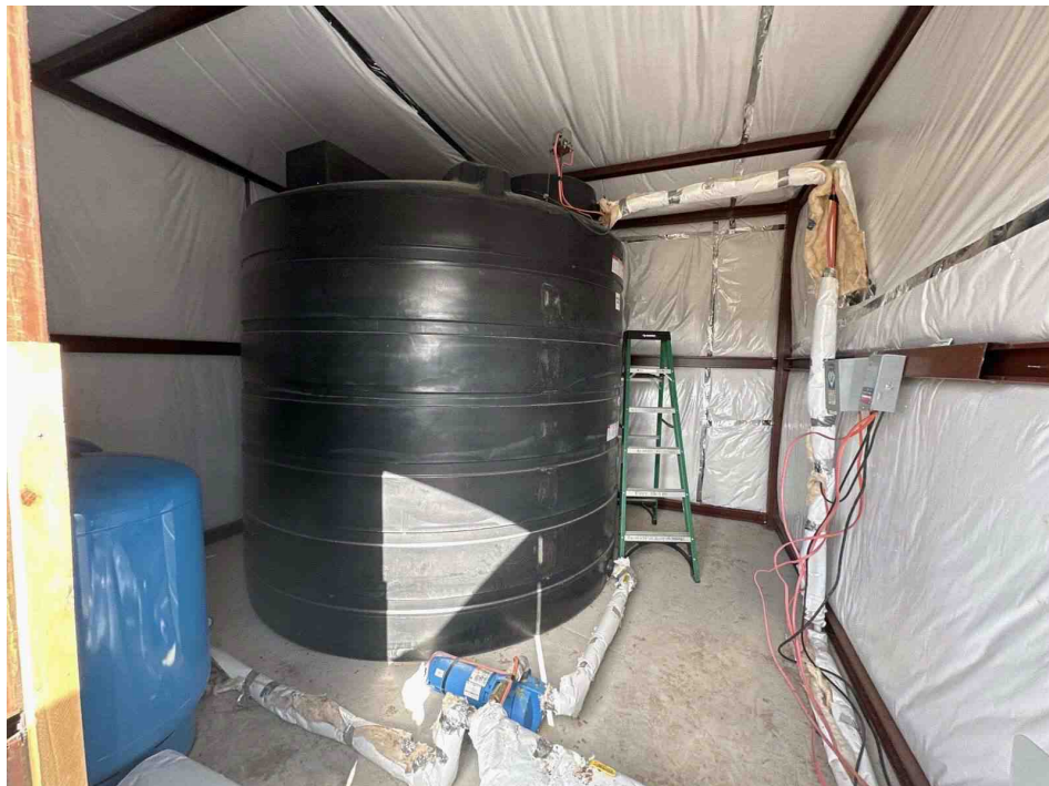
Storage Shed - Interior
