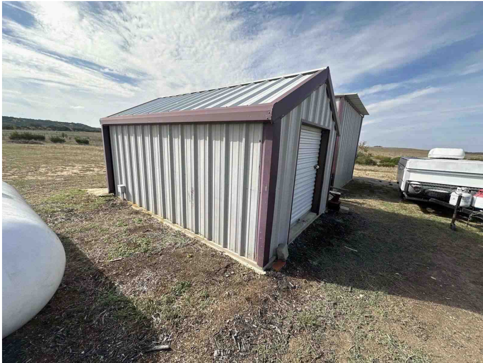
Storage Shed - Exterior
