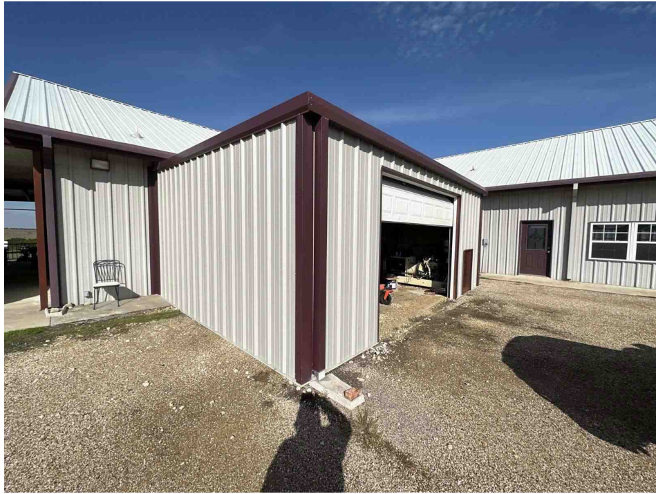
Work Shop - Exterior
