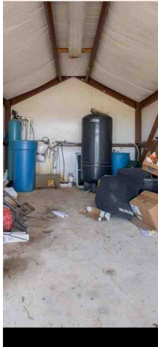
Storage Shed - Interior
