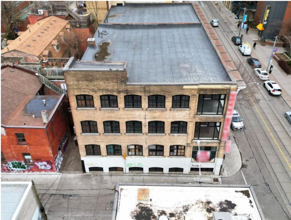
Malabar Building has a laneway at the west side of the building.
