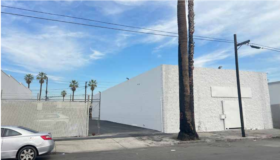
Front of Building
