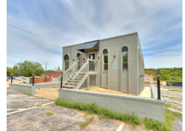
West exterior to suite A and parking.
