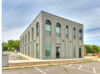
East exterior entrance to suite B.
