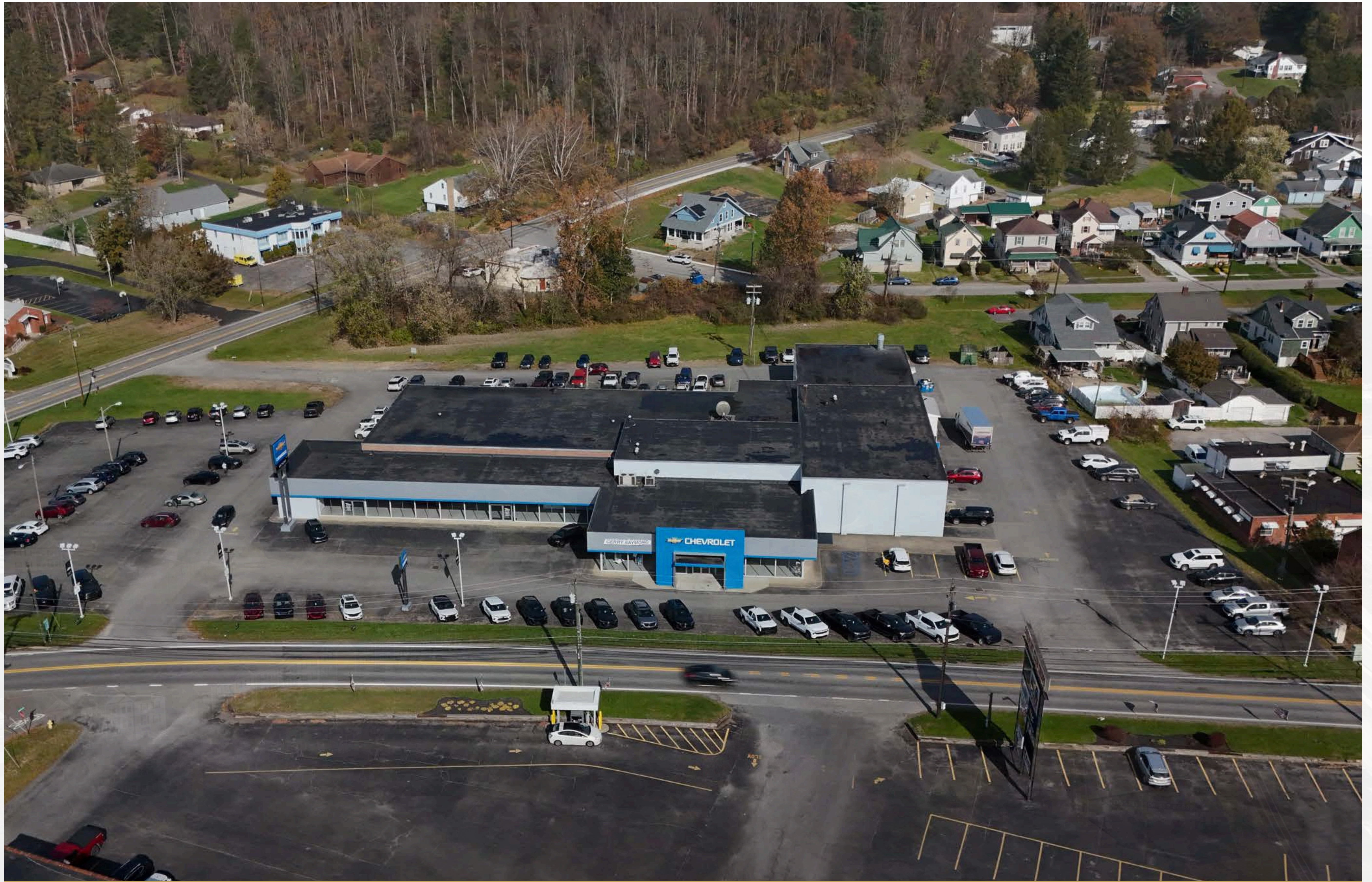
FRONT AERIAL VIEW
