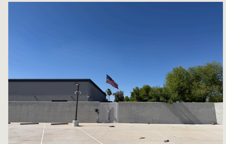
Fig. 02 · 8' CMU wall & vehicle gate
