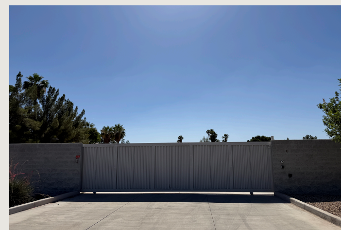
Fig. 03 · Primary motorized access gate
