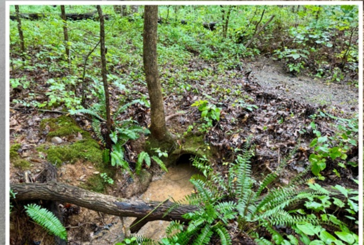
DRIVEWAY CULVERT IN PLACE
