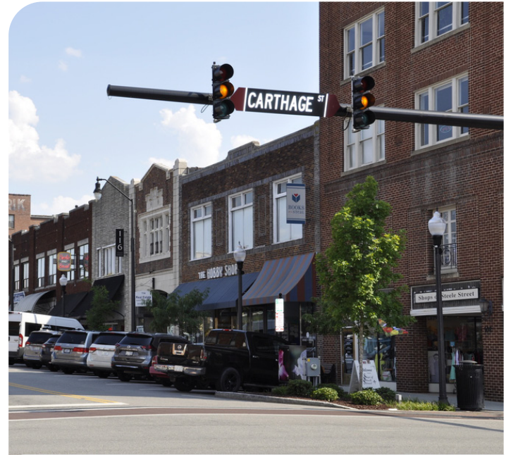
VIEW ALONG S STEELE STREET
