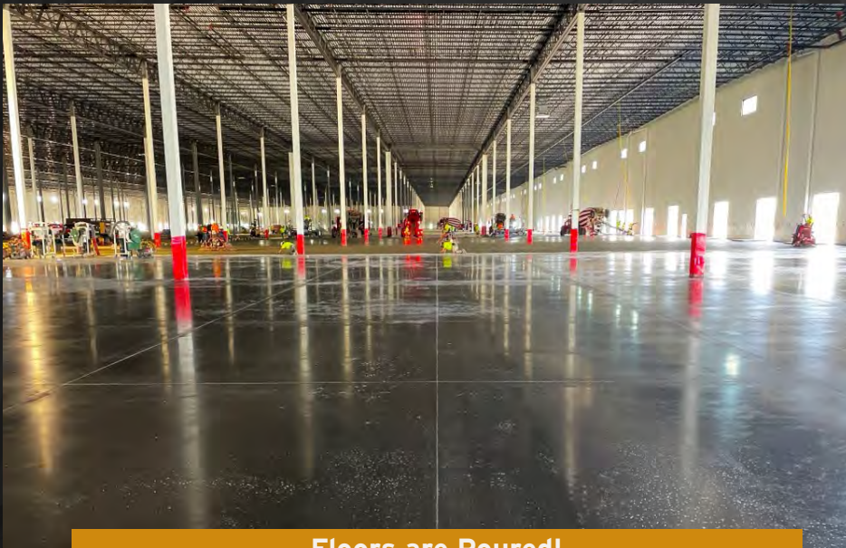
Floors are Poured!
