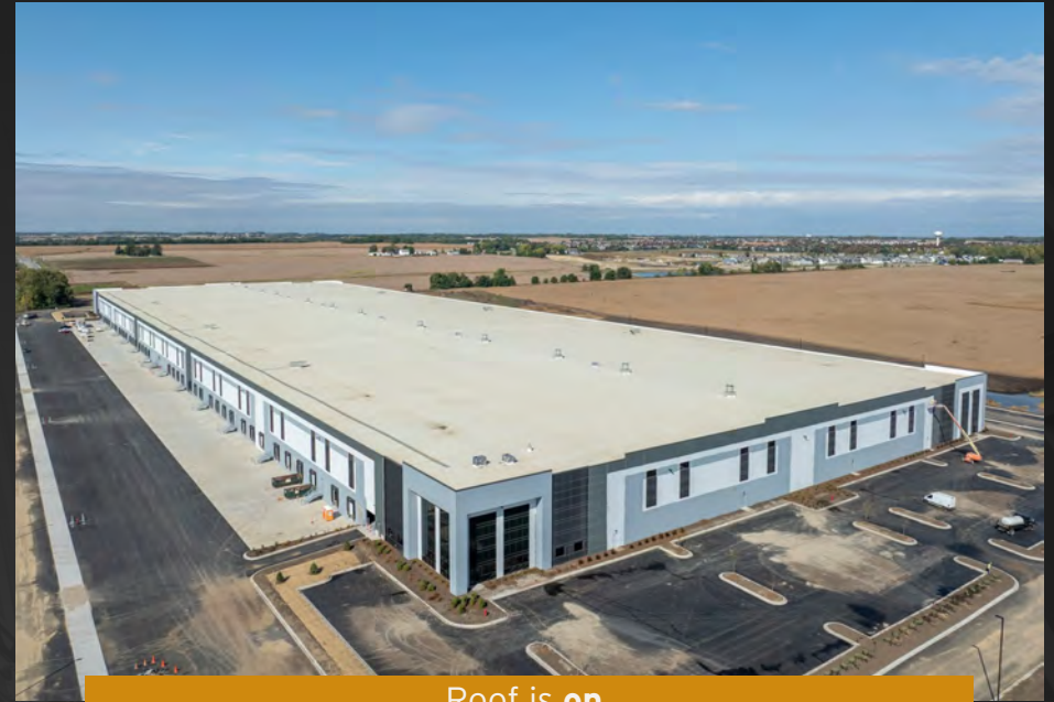
Roof is on.
