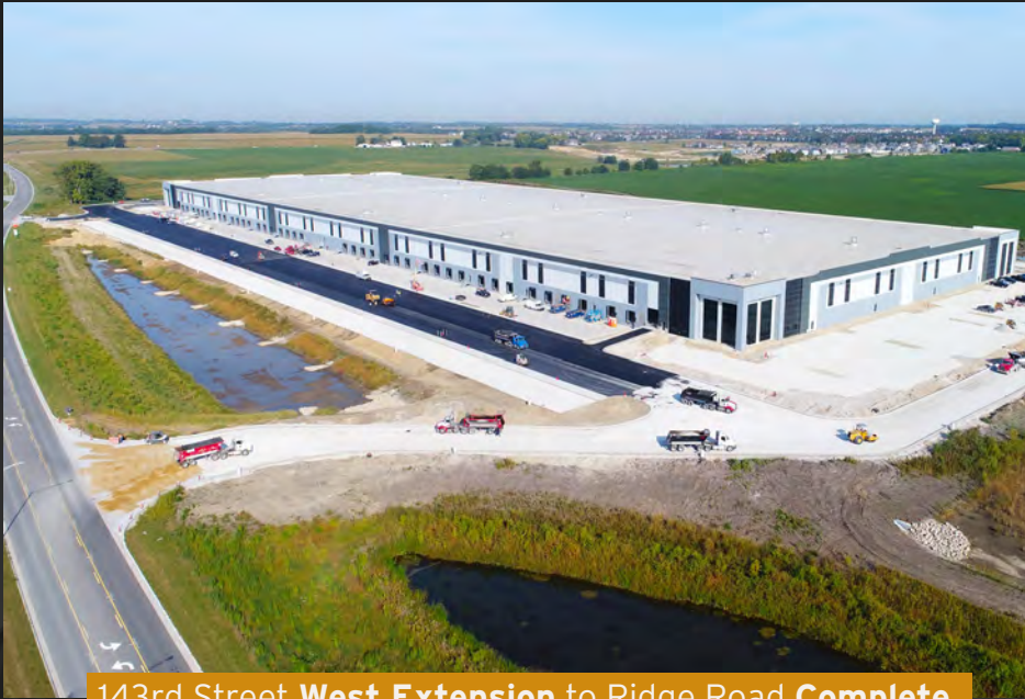
143rd Street West Extension to Ridge Road Complete.
