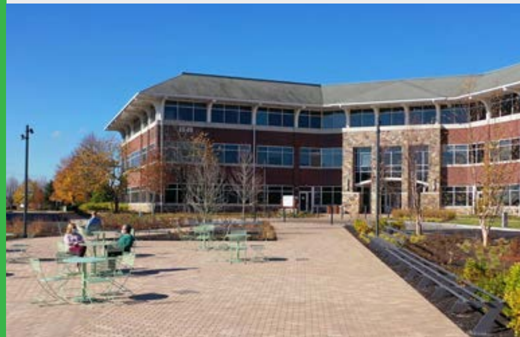
A new outdoor plaza becomes a social hub and gathering place for dining, meeting space, and collaboration.
