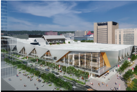
Convention Center Renovation Full Office Renovation
