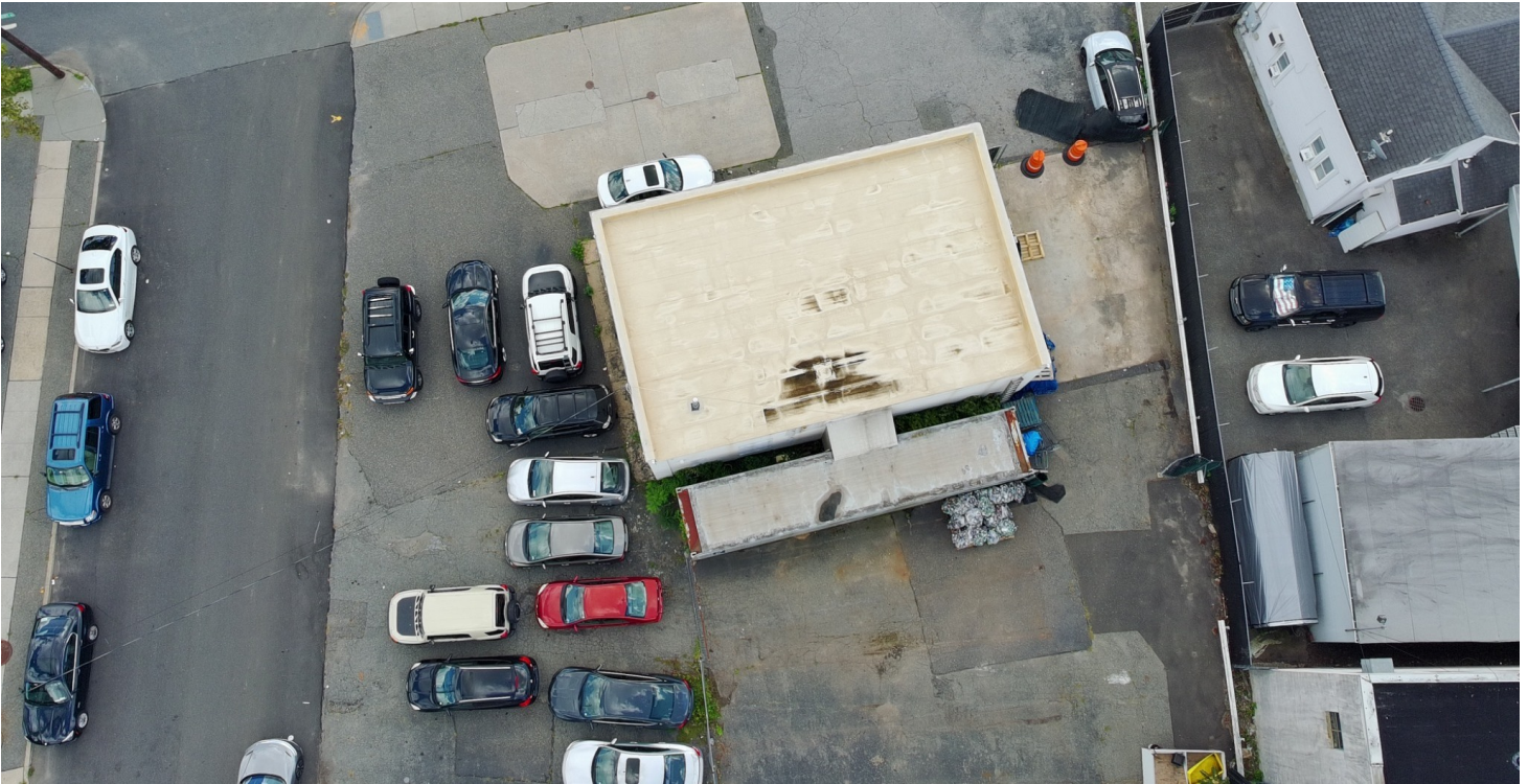
CURRENT OVERHEAD AERIAL
