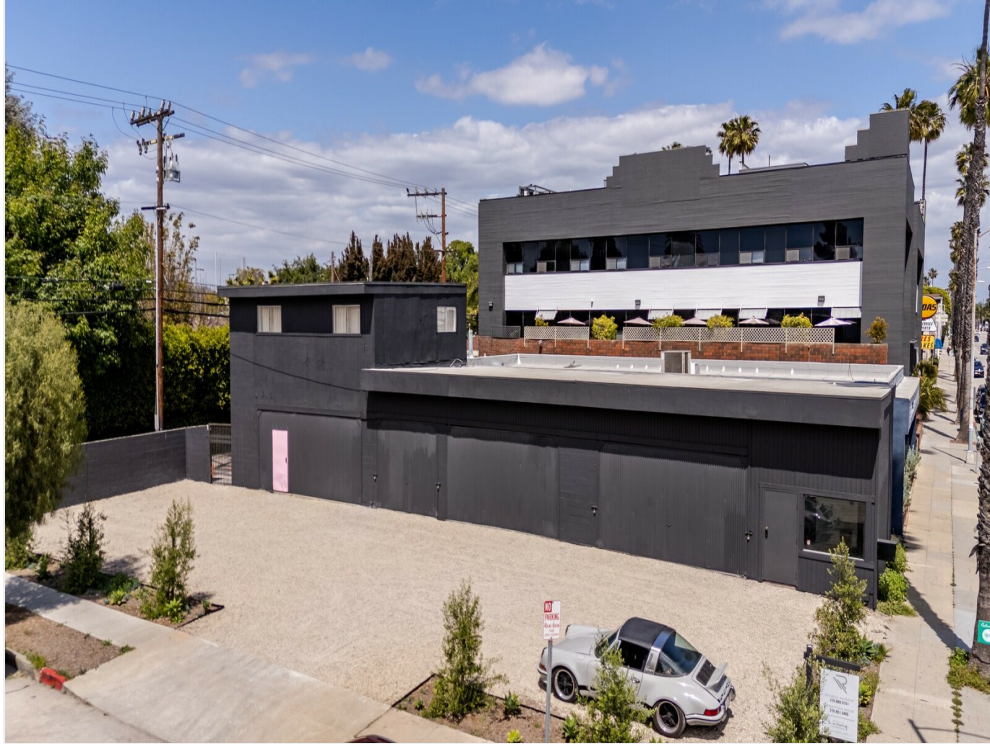
Front of building bays closed
