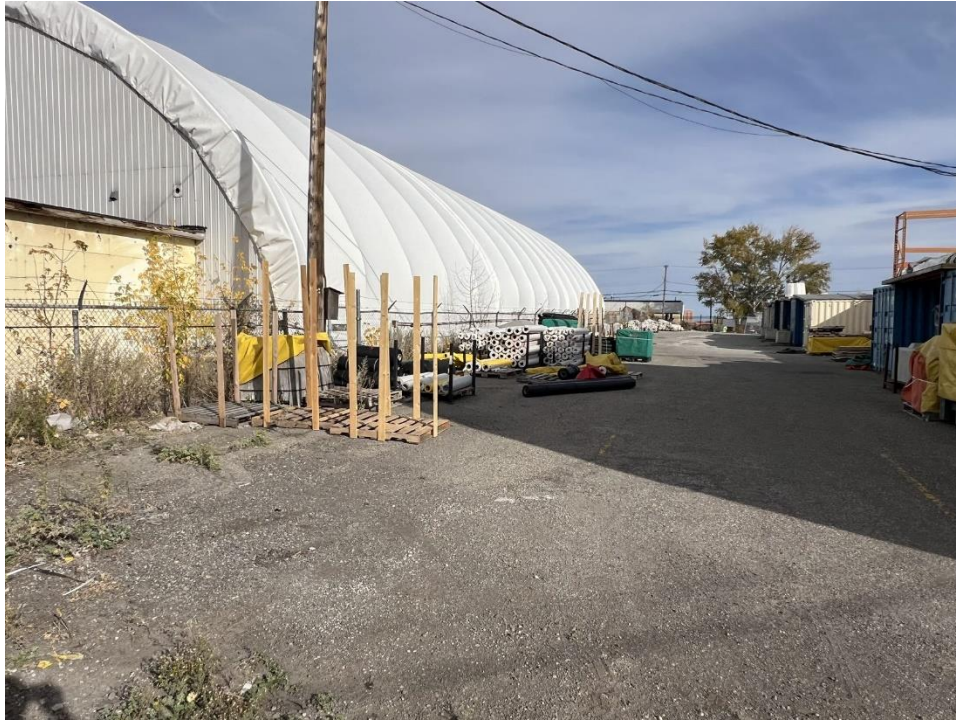
Interior Driveway towards east
