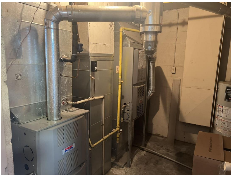
Furnace Room 1 – Workshop Level
