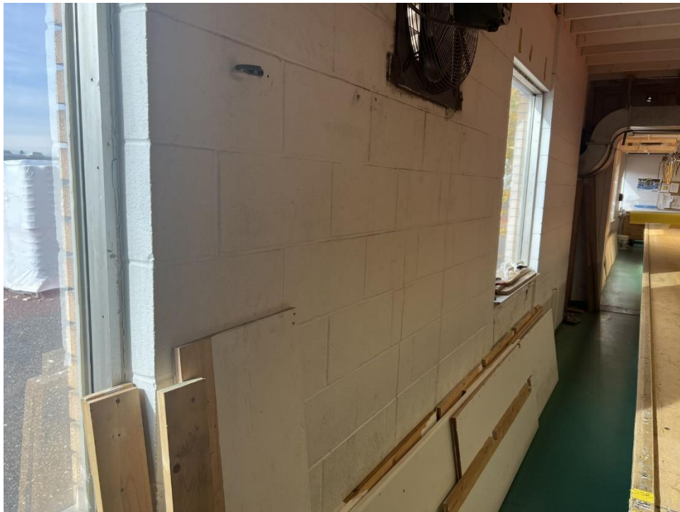
Exterior Concrete Block Wall
