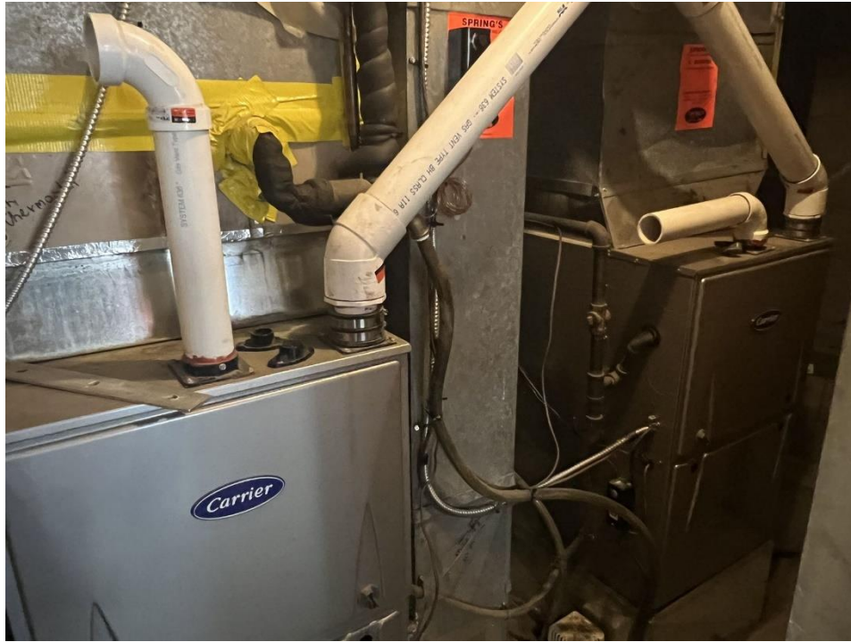
Furnace Room 2 – Main Floor
