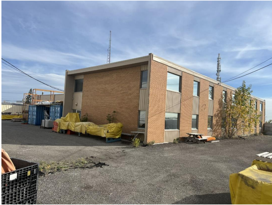
View of the building towards southeast
