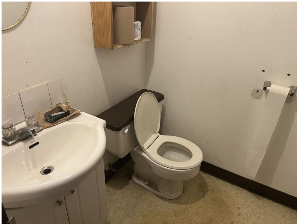
Bathroom – Workshop Level
