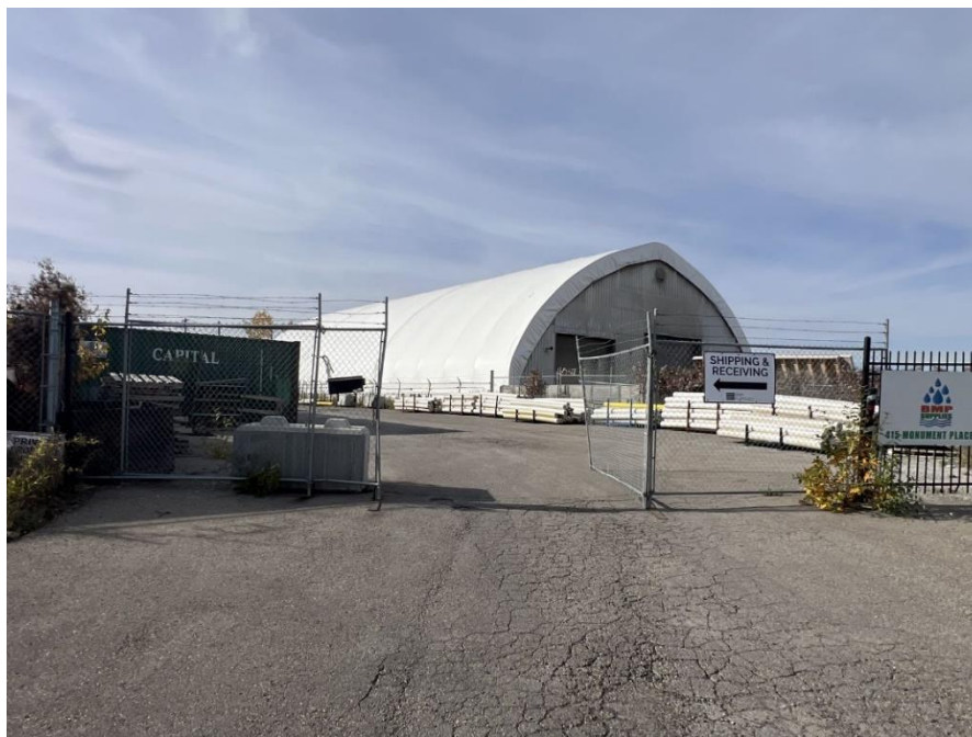
2 nd Entrance of the subject towards northeast
