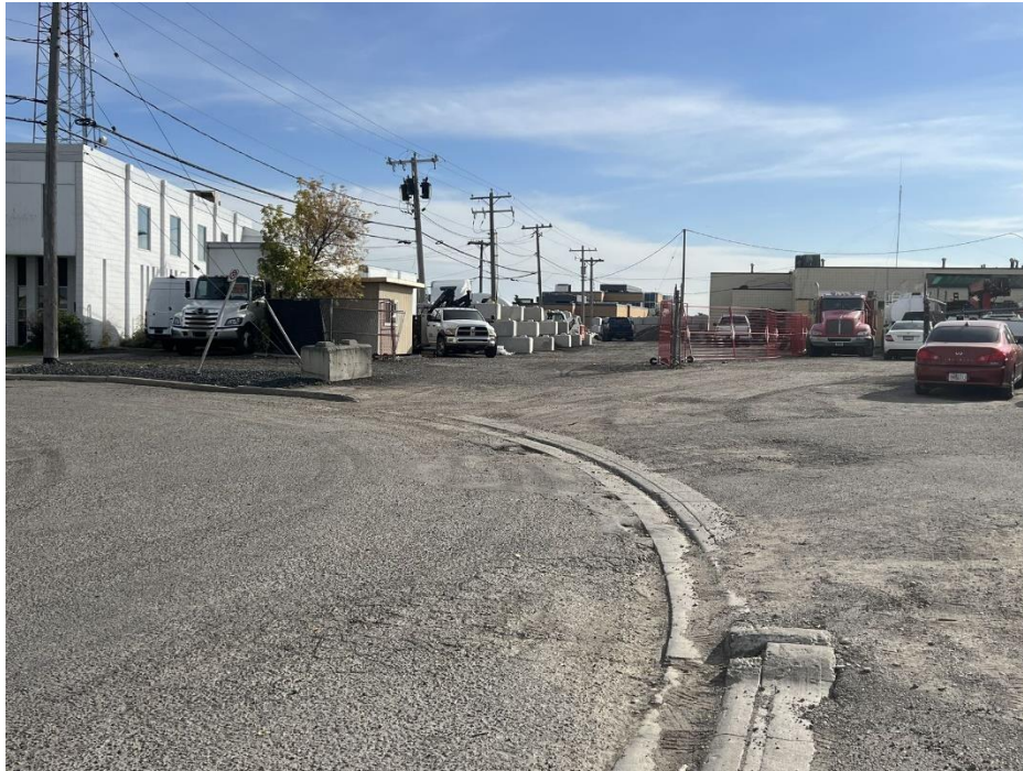
Street View towards east
