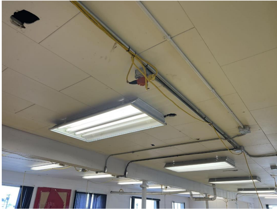
Ceiling – Upper Floor
