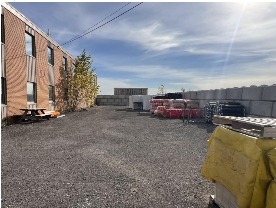
Back loading yard to the west
