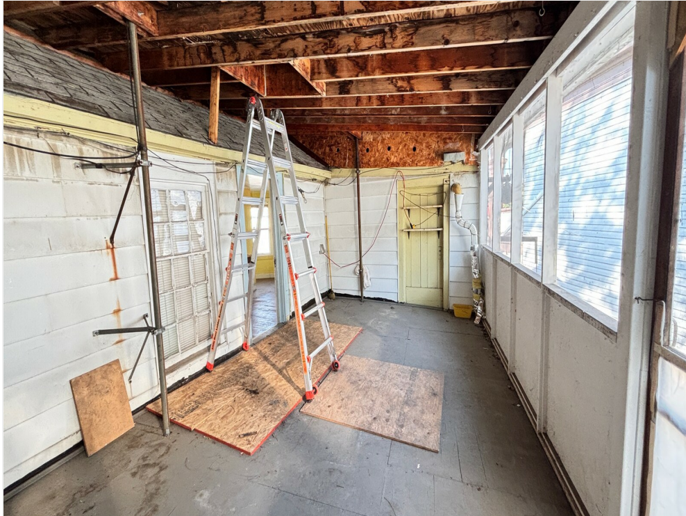
2nd Fl - Apt A - Side Porch (off Kitchen)
