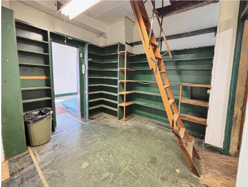
1st Fl - Stockroom A-Side - with Stairs to Apartment B/Now Storage
