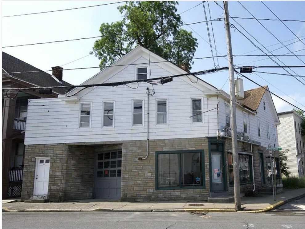
Exterior - Columbia St Side
