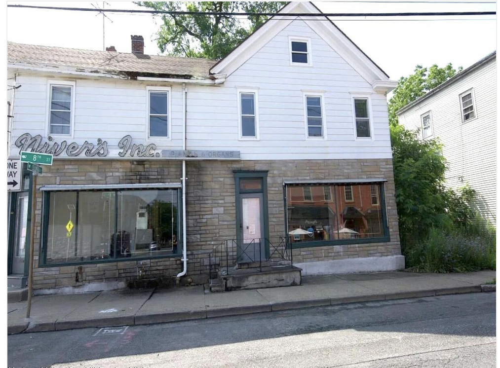
Exterior - 8th St Side
