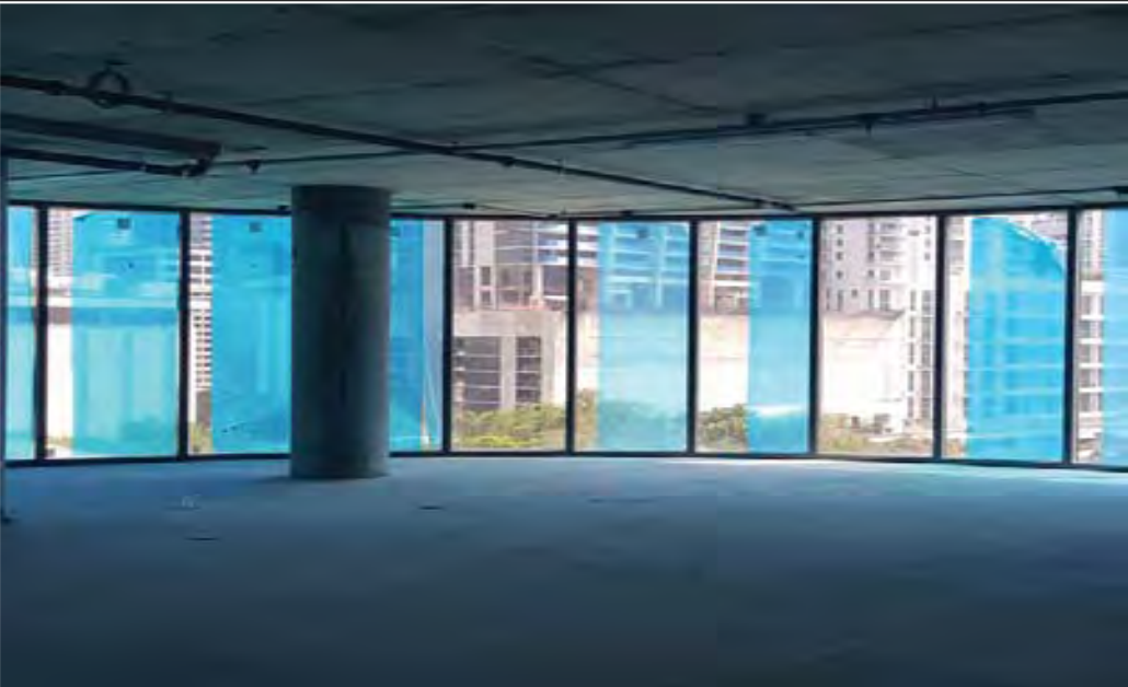
CORNER UNIT AREA VIEW
