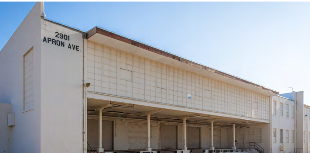
Ground-Level View: Dock-High Doors
