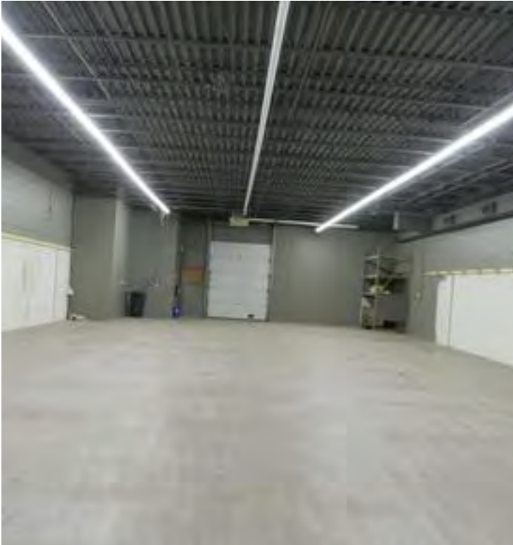
Main section of retail space showing inside of loading dock
