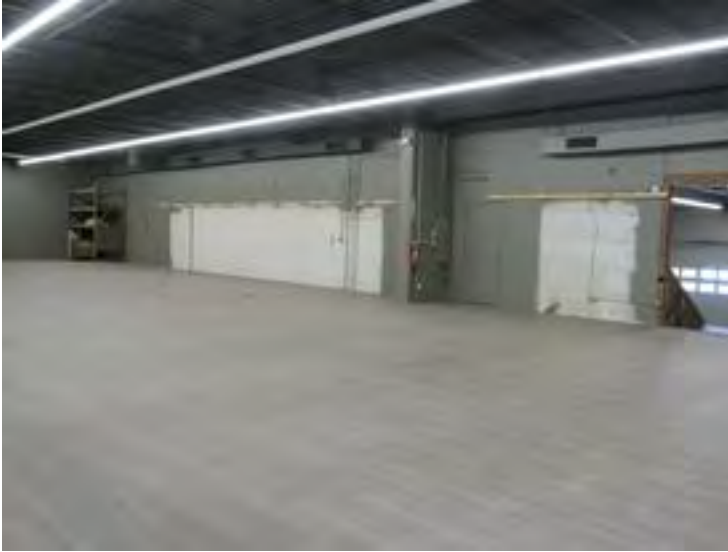
Side view of large retail space
