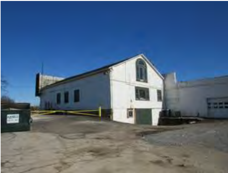
Side view of office retail section
