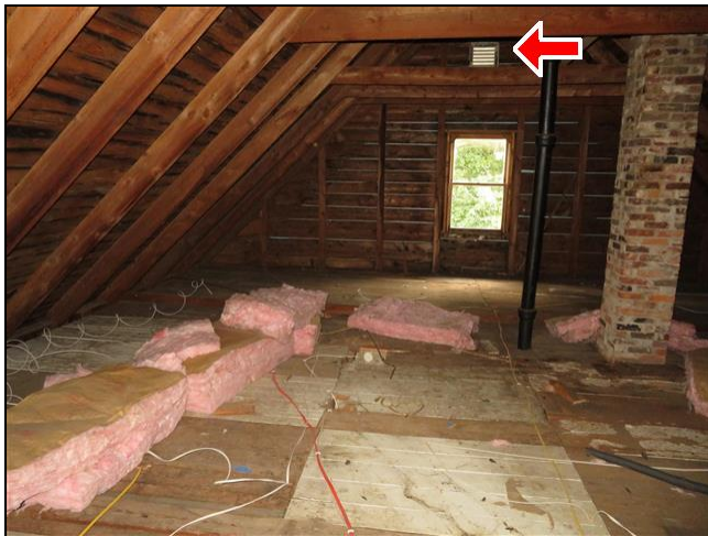
9.3 Item 1(Picture) Attic
