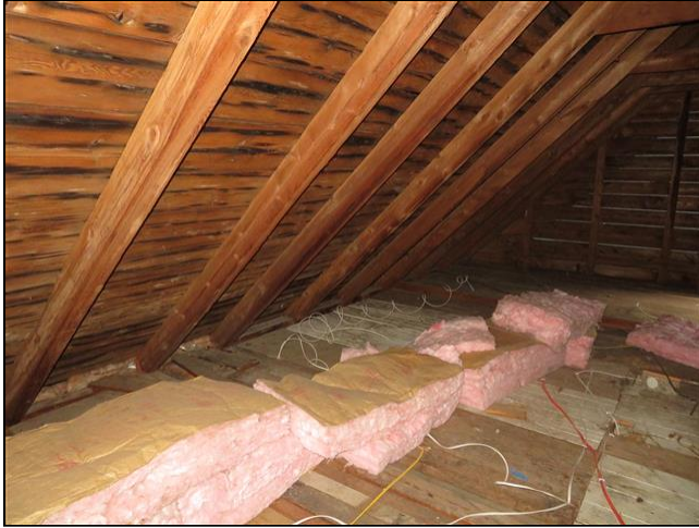
5.9 Item 1(Picture) Attic
