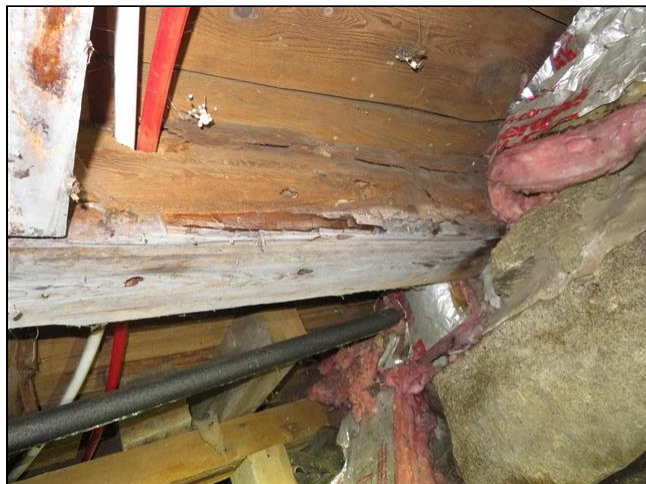
5.5 Item 5(Picture) Crawlspace
