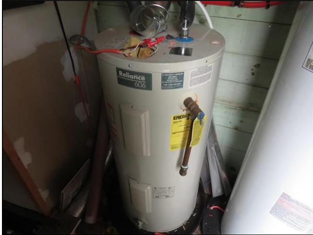
4.10.B Item 1(Picture) Utility room
