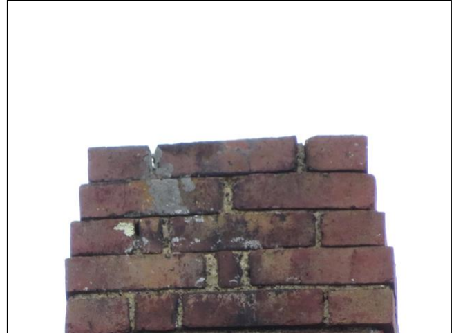
2.3 Item 11(Picture) Right side chimney
