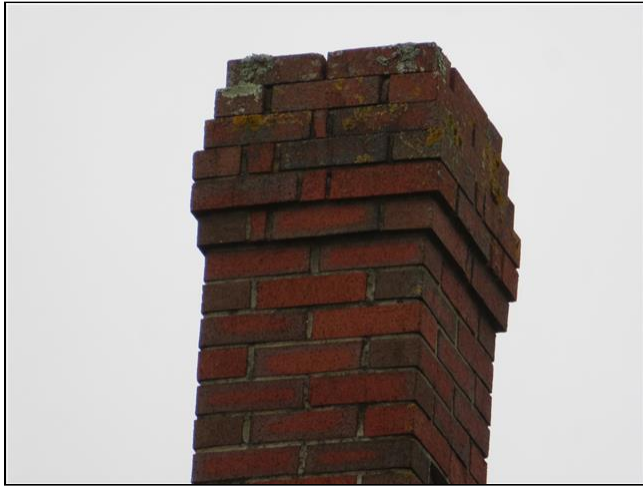
2.3 Item 5(Picture) Left side chimney
