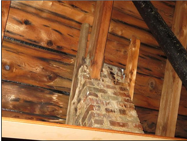
5.7 Item 3(Picture) Attic
