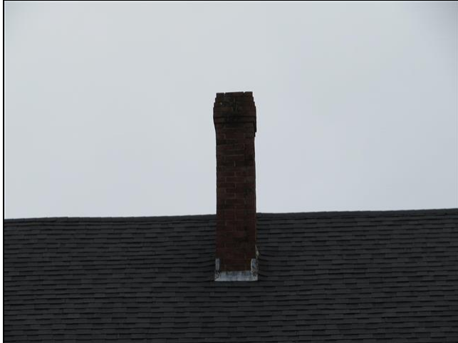
2.3 Item 10(Picture) Right side chimney
