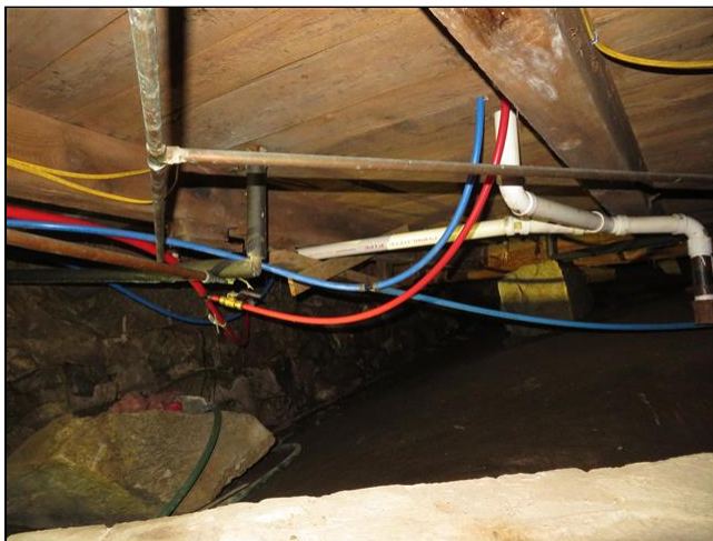
6.1 Item 1(Picture) Crawlspace
