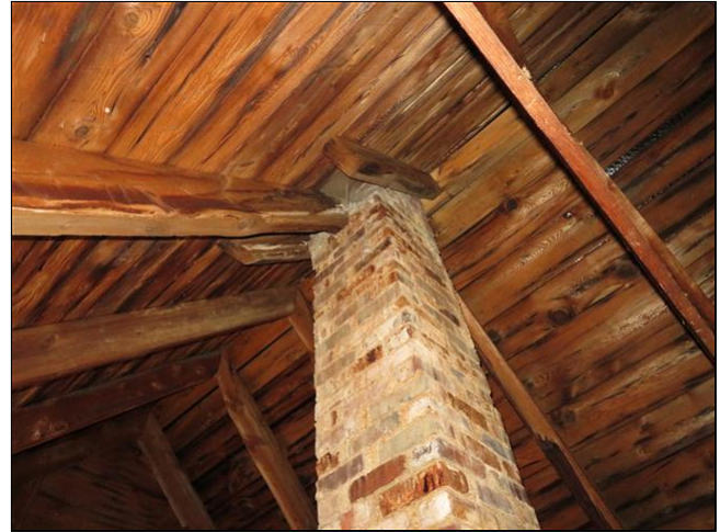
5.7 Item 4(Picture) Attic
