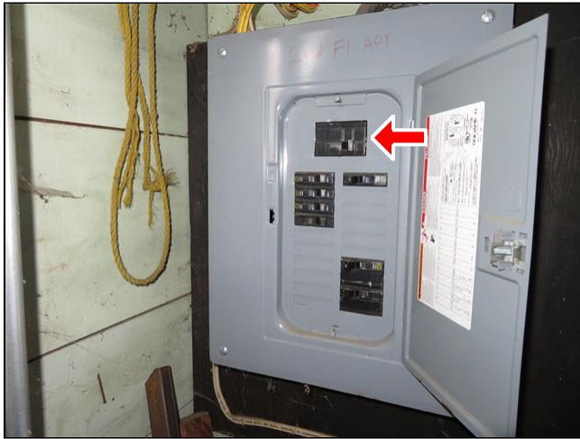
4.14.B Item 1(Picture) Attached garage
