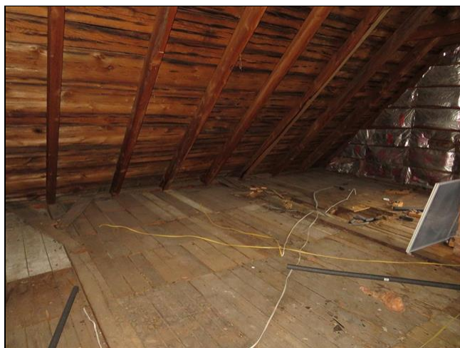
5.7 Item 1(Picture) Attic
