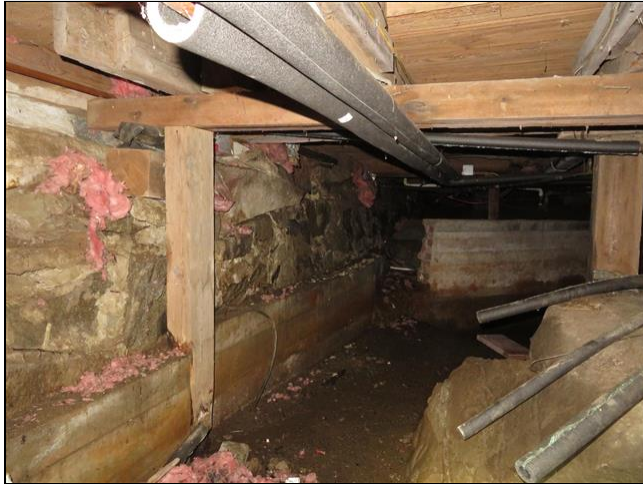
5.4 Item 1(Picture) Crawlspace
