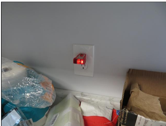
4.17.B Item 1(Picture) Kitchen
