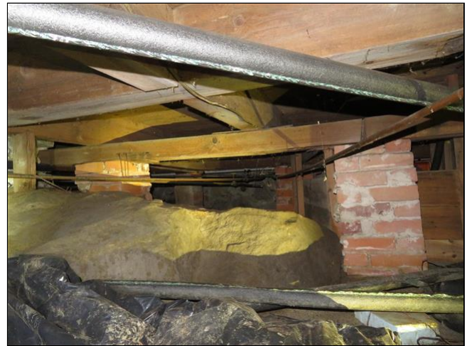
5.1 Item 5(Picture) Crawlspace
