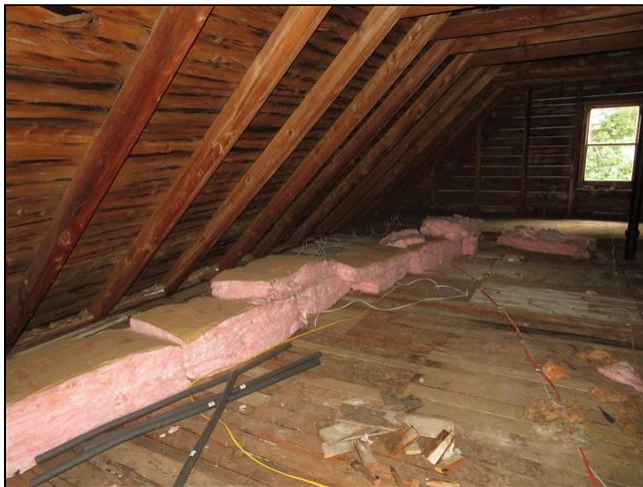
5.8 Item 1(Picture) Attic
