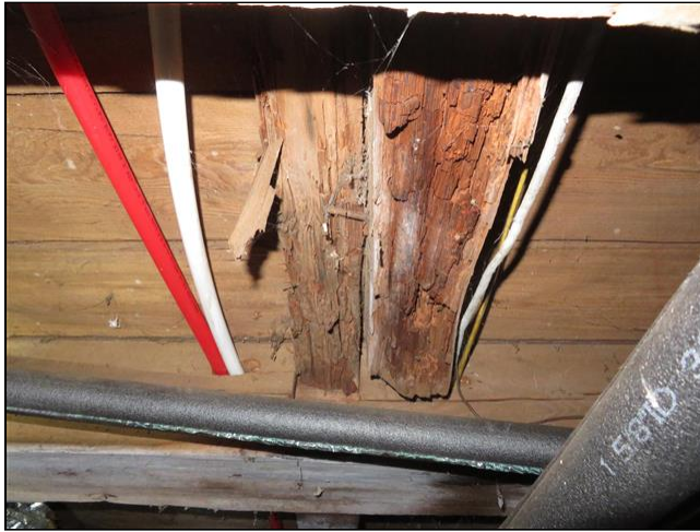
5.5 Item 1(Picture) Crawlspace
