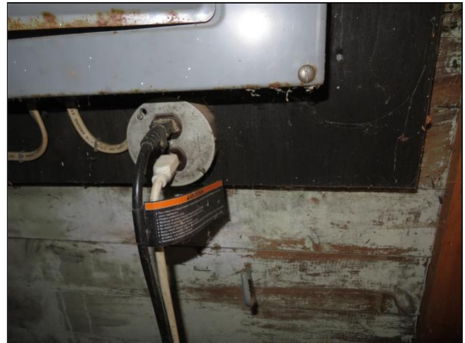
7.4 Item 2(Picture) Attached garage
