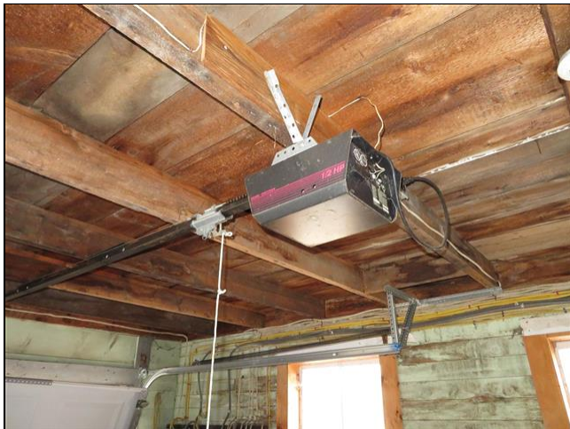
3.8 Item 1(Picture) Attached garage
