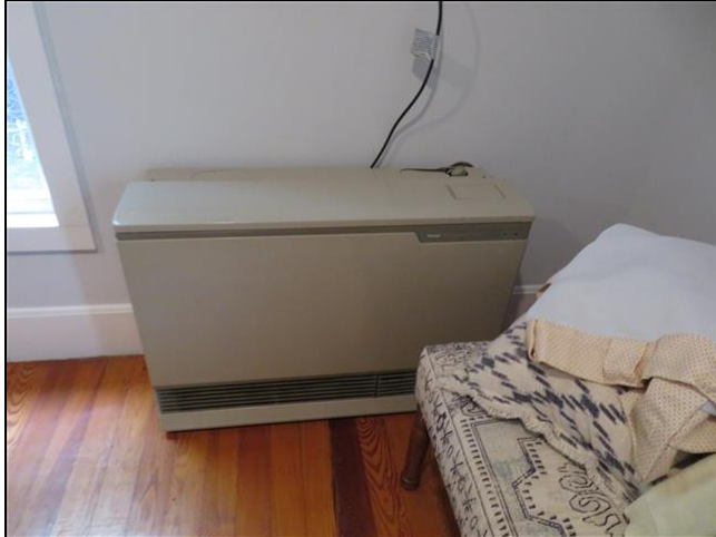
4.23.B Item 2(Picture) Living room
