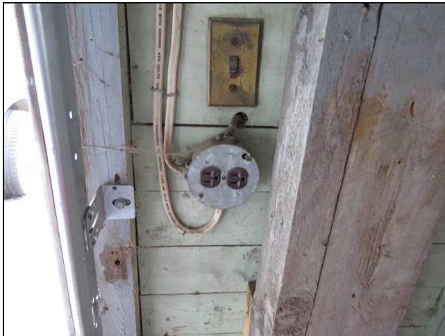
7.4 Item 1(Picture) Attached garage
