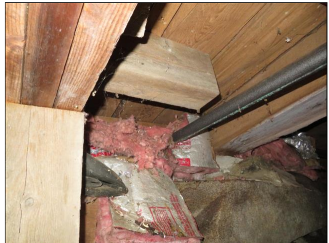
5.1 Item 8(Picture) Basement
