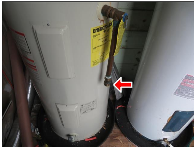
4.10.B Item 2(Picture) Utility room
