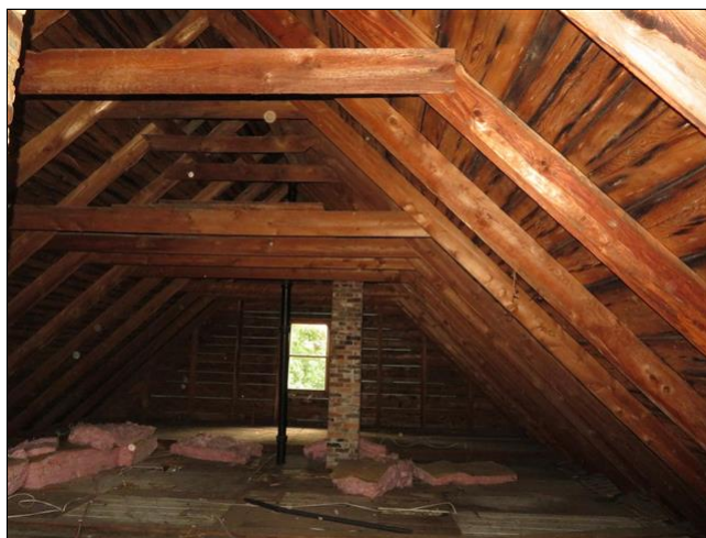
5.7 Item 2(Picture) Attic
