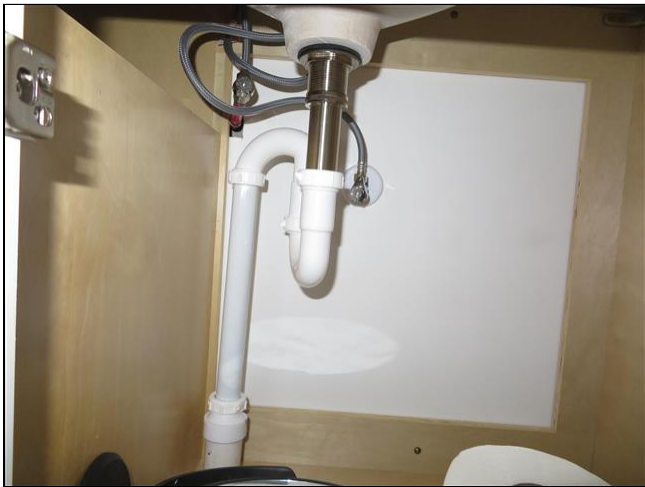
4.8.B Item 1(Picture) Bathroom
