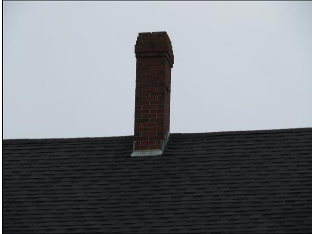
2.3 Item 1(Picture) Left side chimney
