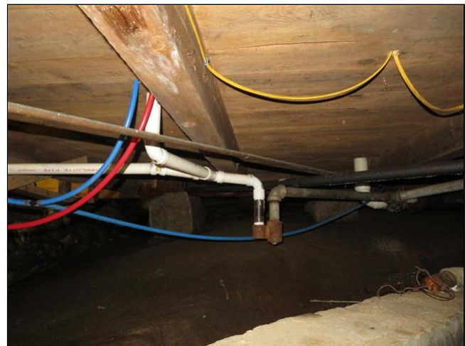
6.1 Item 2(Picture) Crawlspace
