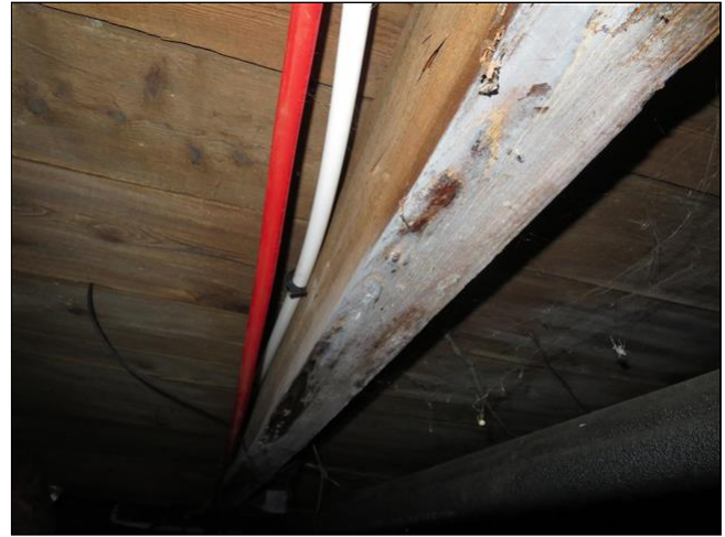
5.5 Item 2(Picture) Crawlspace
