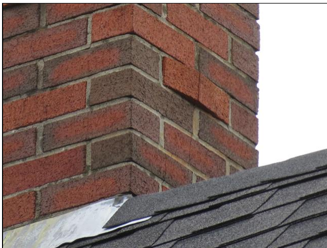
2.3 Item 9(Picture) Left side chimney
