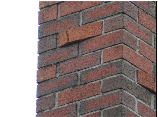
2.3 Item 8(Picture) Left side chimney
