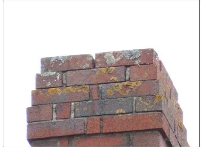
2.3 Item 2(Picture) Left side chimney
