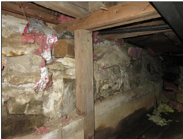
5.3 Item 1(Picture) Crawlspace
