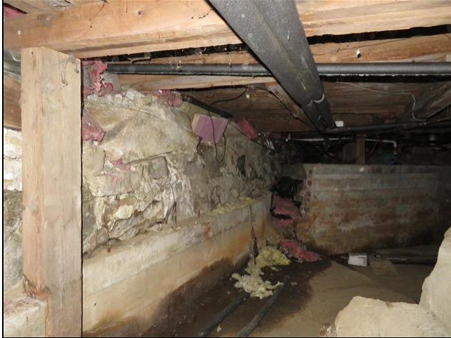
5.1 Item 3(Picture) Crawlspace
