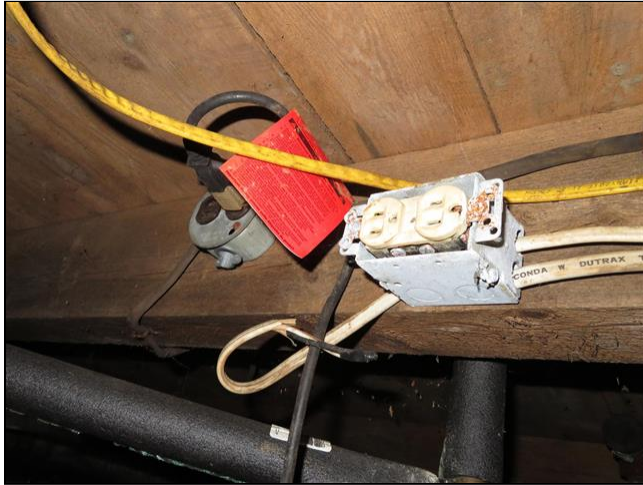
7.4 Item 3(Picture) Crawlspace
