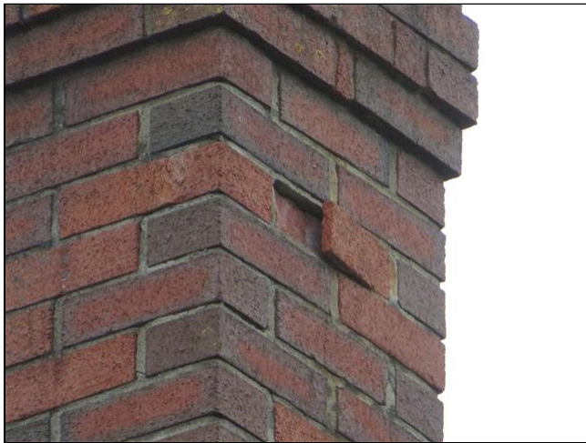
2.3 Item 7(Picture) Left side chimney
