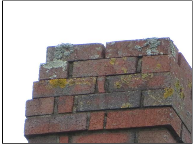
2.3 Item 6(Picture) Left side chimney
