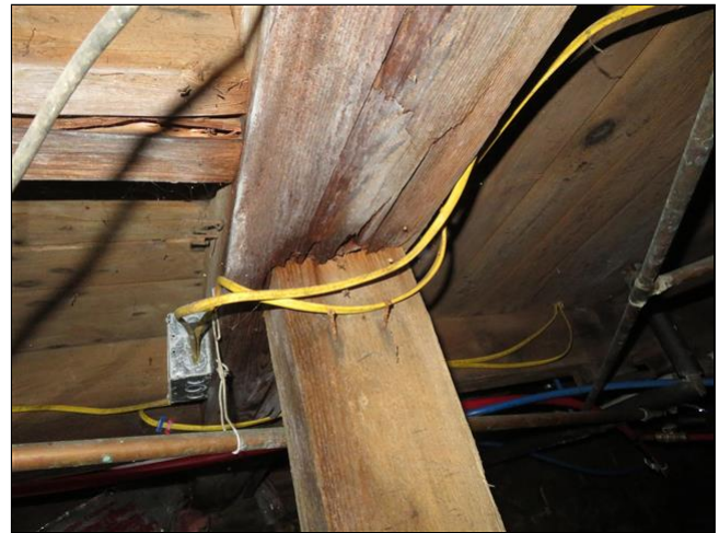
5.5 Item 4(Picture) Crawlspace
