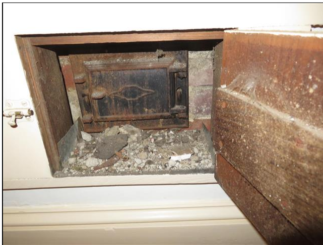
8.0 Item 7(Picture) Right side chimney
