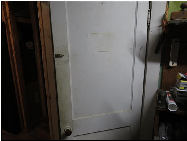
3.7 Item 1(Picture) Attached garage
