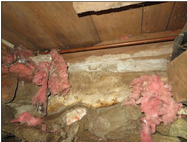
5.1 Item 7(Picture) Basement
