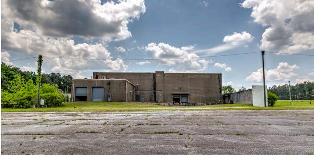
NORTH WALL - 2 GRADE LEVELS AND TWO DOCK HIGHS
