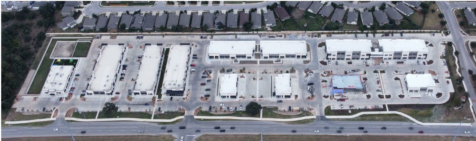
CONSTRUCTION PROGRESSION AS OF SEP 2024
