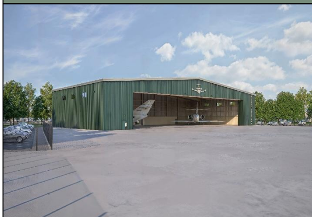
Republic Airport | Farmingdale, NY 387k SF hangar development
