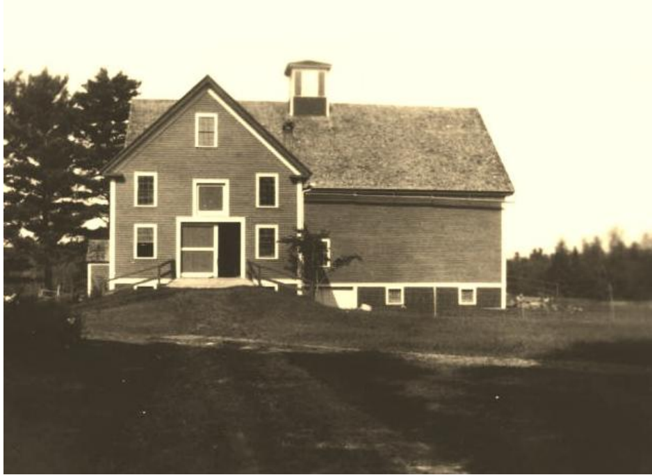
Photo of the Twitchell barn showing on the right (north) end the gradual sloped bridge made to allow horse to pull loaded hayracks into the barn.
