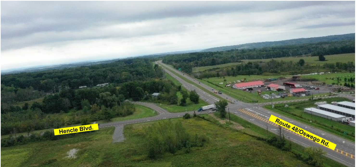
Facing South – Hencle Blvd curb cut and 4-way lighted intersection
