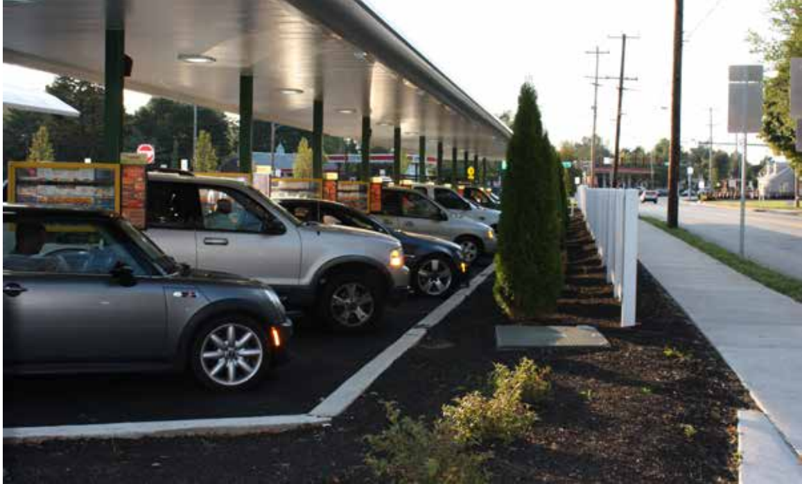
Figure 24.4 Parking Lot Screen
