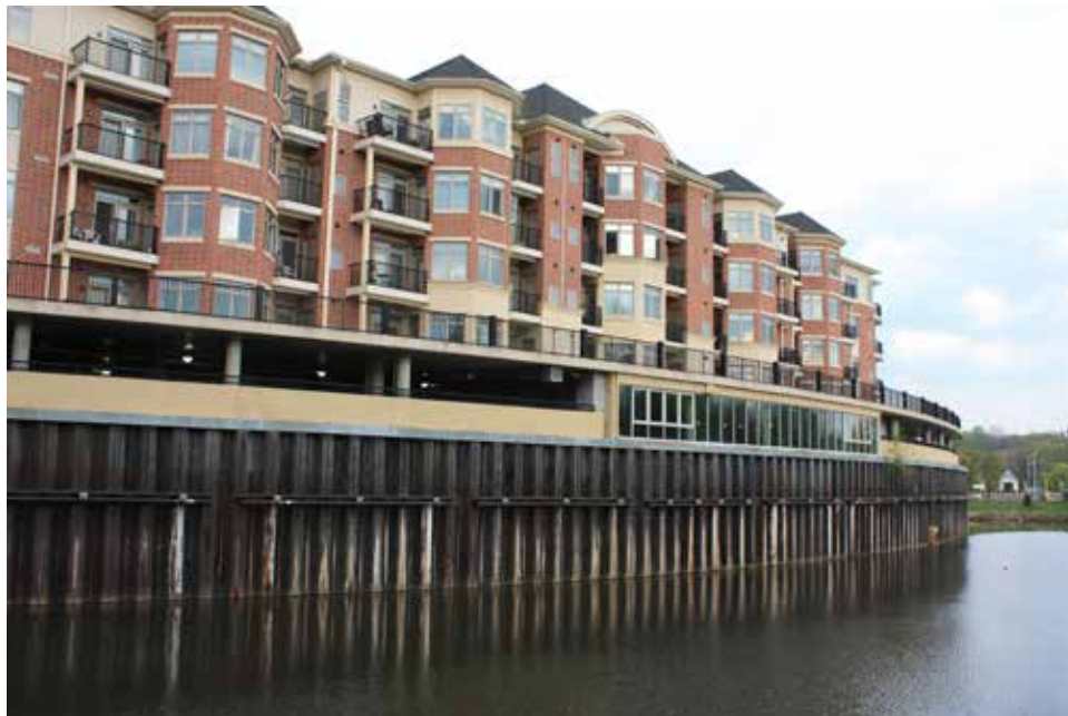
Elevated Structure, Pennypack Creek
