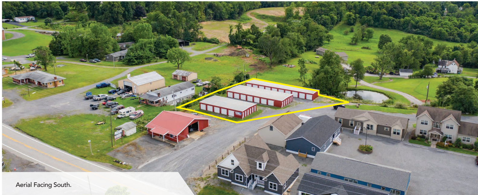
Aerial Facing North.
