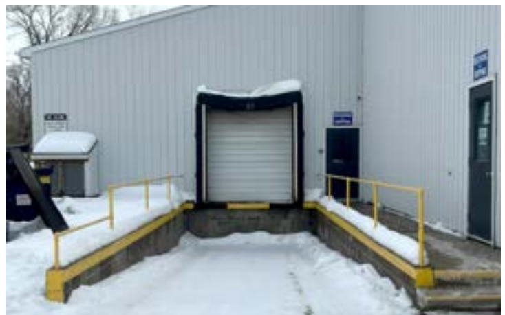
Truck Dock With 8'W x 8'9"H Overhead Door
