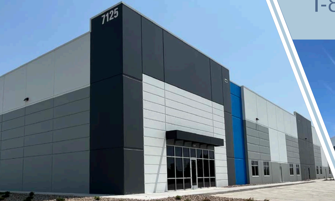
I-35 DISTRIBUTION CENTER 7055 - 7125 SE DELAWARE, ANKENY, IA
