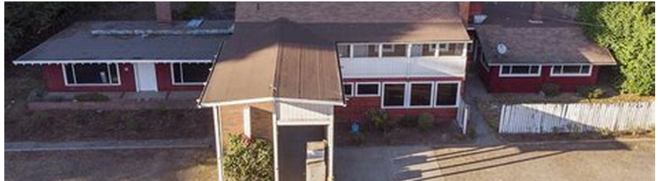
INN BUILDING — AERIAL
