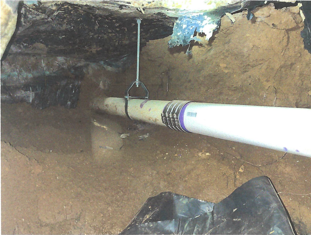
New plumbing connects to existing outside of grade beams
