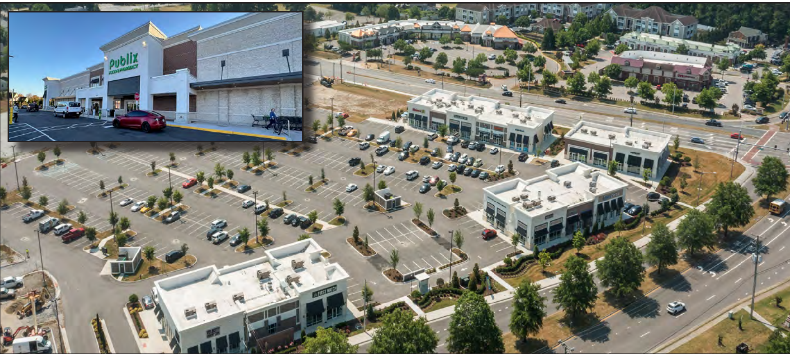
Hickman Place | 2160 - 2218 General Booth Blvd., Virginia Beach, VA
