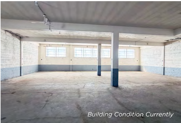
Building Condition Currently
