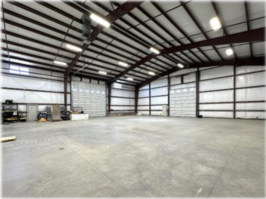
A-6 – South Side of Building A
