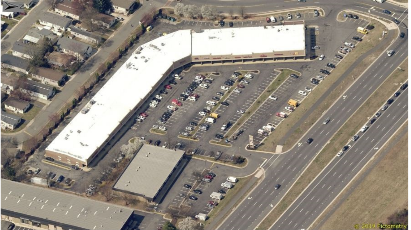
Figure 2103.15: C-8 District Aerial Example
