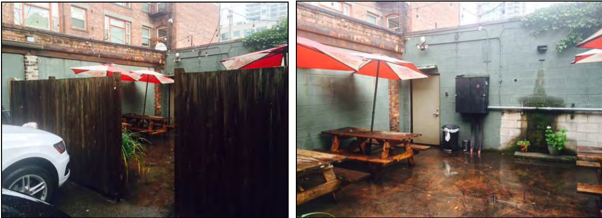
Above left, looking northeast at the fence that subdivides the courtyard and back patio with portions of the primary building section (right) and the north wing (left). The Fleming Apartment building is visible in the background.
