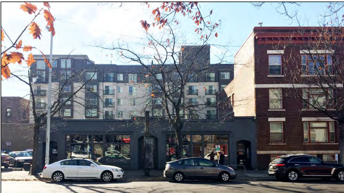
Below, looking west at the primary east façade in November 2017.
