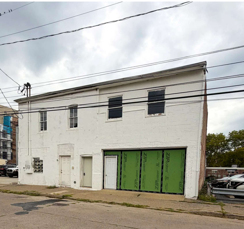
211 Mechanic St - Front View
