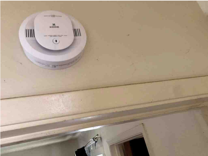
SMOKE & CO DETECTOR/UNIT A
