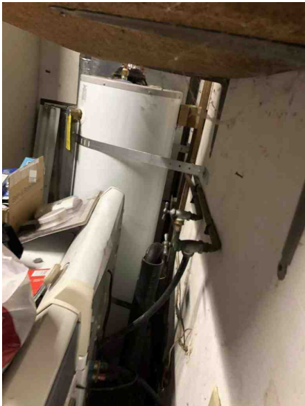
WATER HEATER DOUBLE STRAPPED/UNIT A
