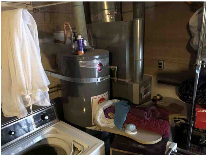
WATER HEATER DOUBLE STRAPPED/UNIT A
