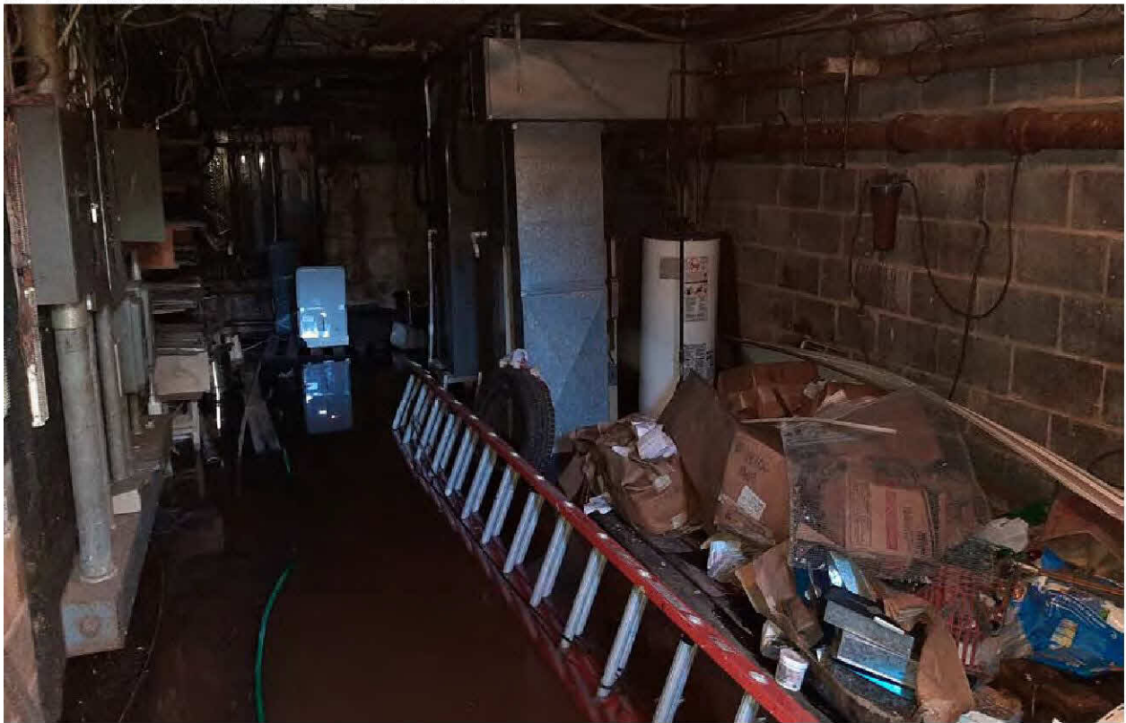
8. View of the basement in the office building.
