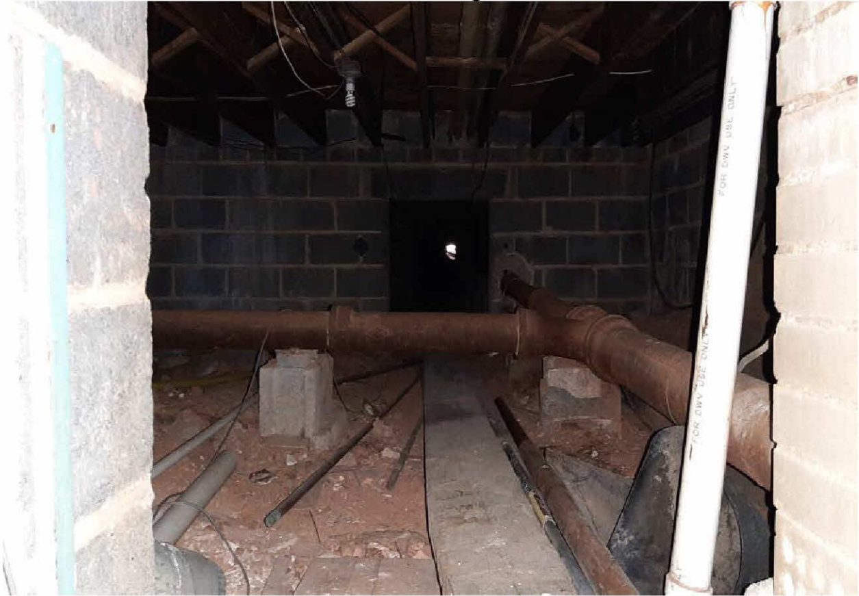
12. View of the basement in one of the motel buildings.
