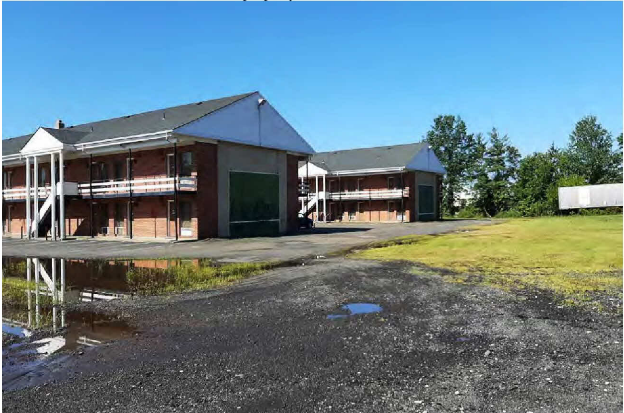
2. View of the exterior of the rear of the property.
