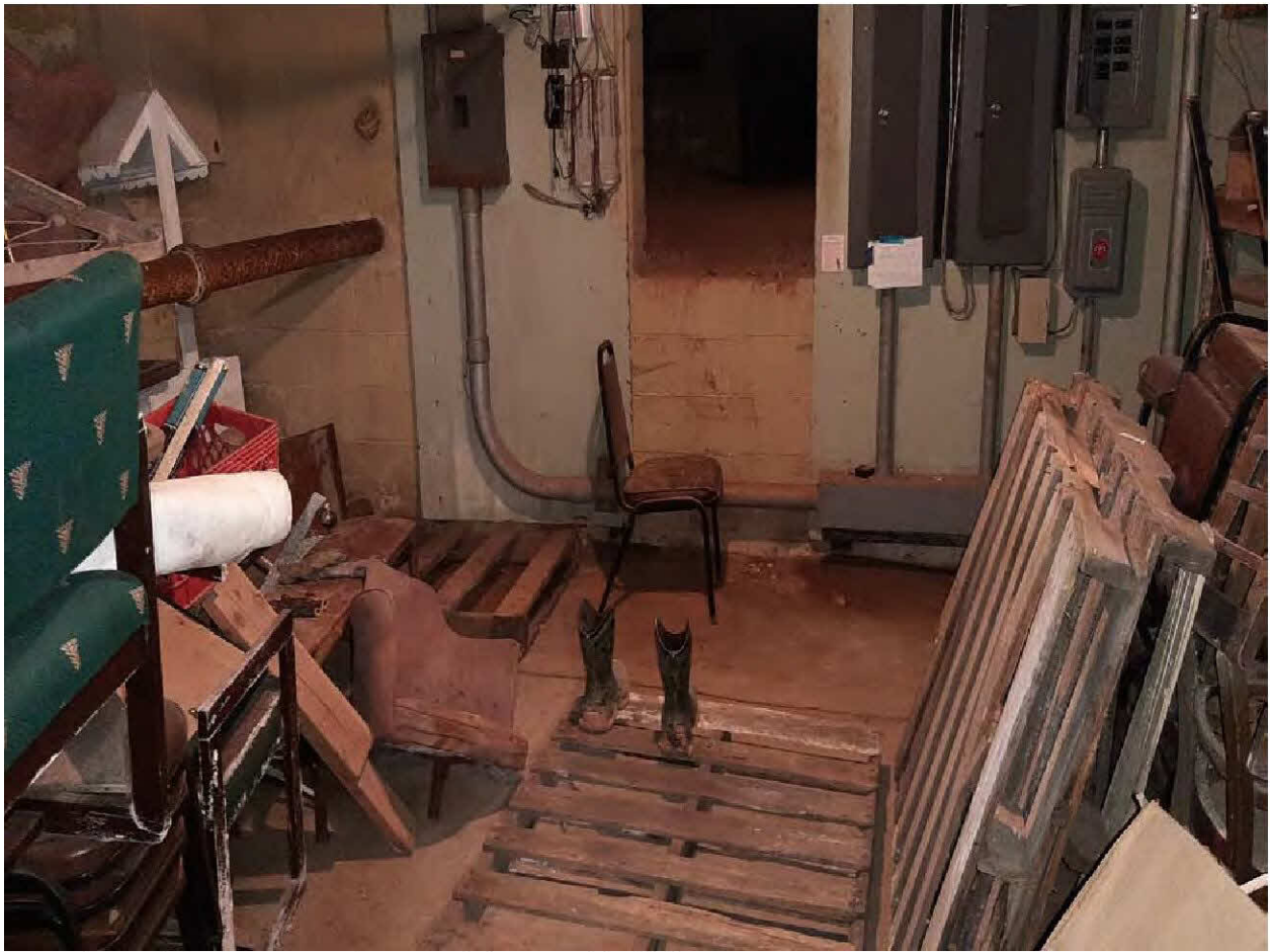
11. View of the basement in one of the motel buildings.
