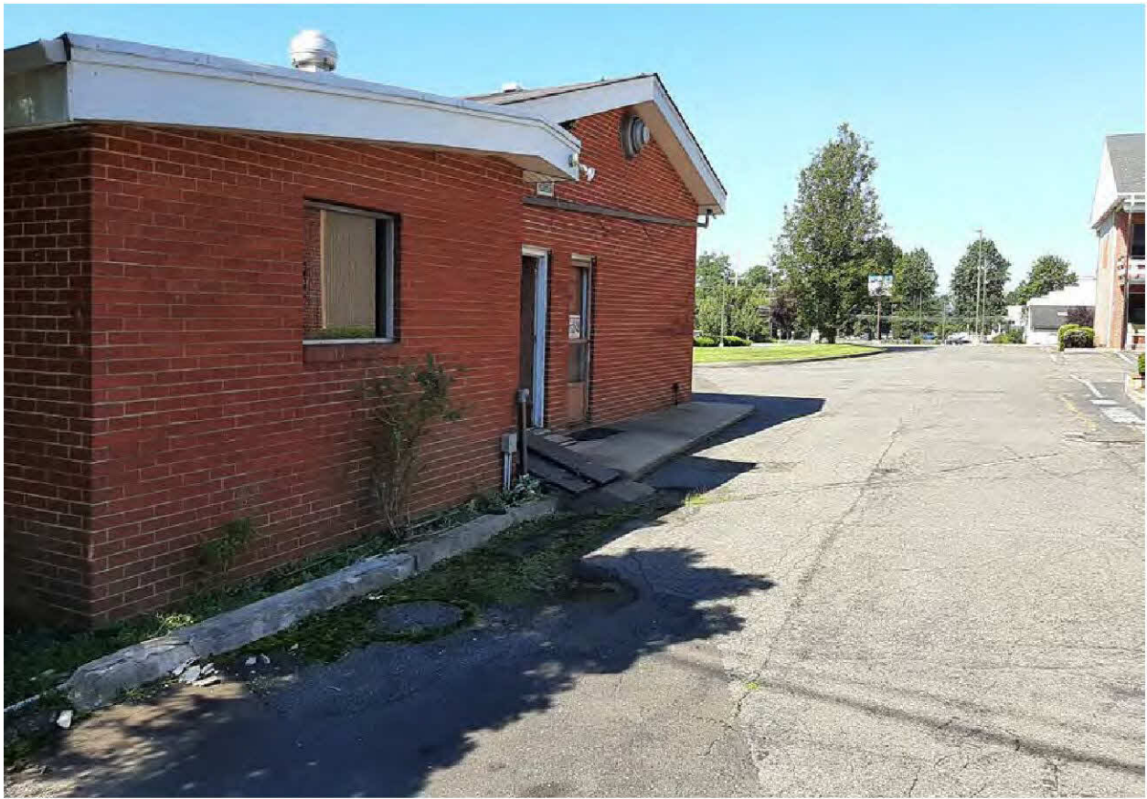
3. View of the exterior of the office building.
