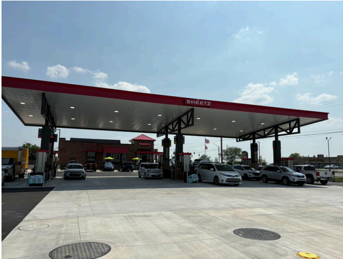
Fuel Canopy & Store Exterior
