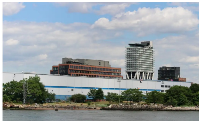
The CitiStorage building at Bushwick Inlet Park, shown in June of this year, is set to be totally demolished by the end of the year. Photo by Susan De Vries
