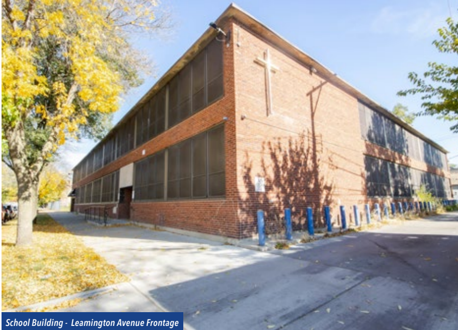
School Building - Leamington Avenue Frontage
