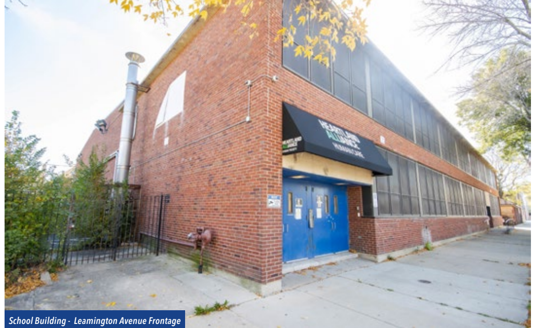
School Building - Leamington Avenue Frontage
