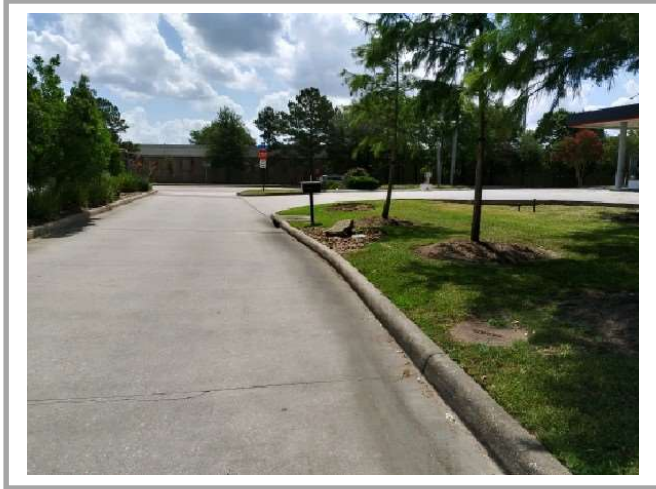
Shenandoah Drive site approach and frontage facing east
