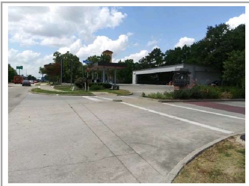
Site view across the intersection of the Interstate 45 southbound frontage road and Shenandoah Drive
