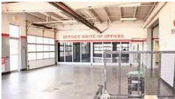
Service reception with write-up offices and overhead doors
