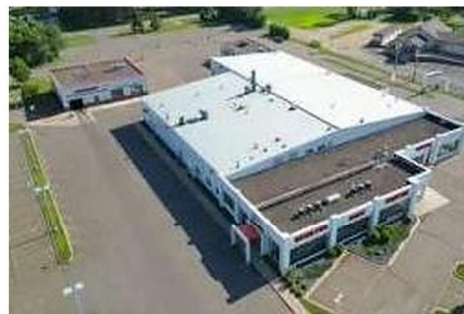
Body shop and rear service doors from the northeast
