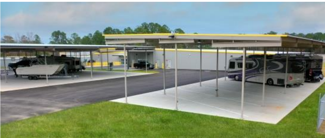
More of Storage King USA's canopy parking
