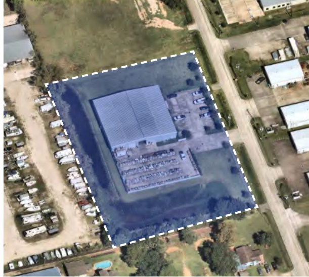
1860 Lawrence Rd Great Western Valve
