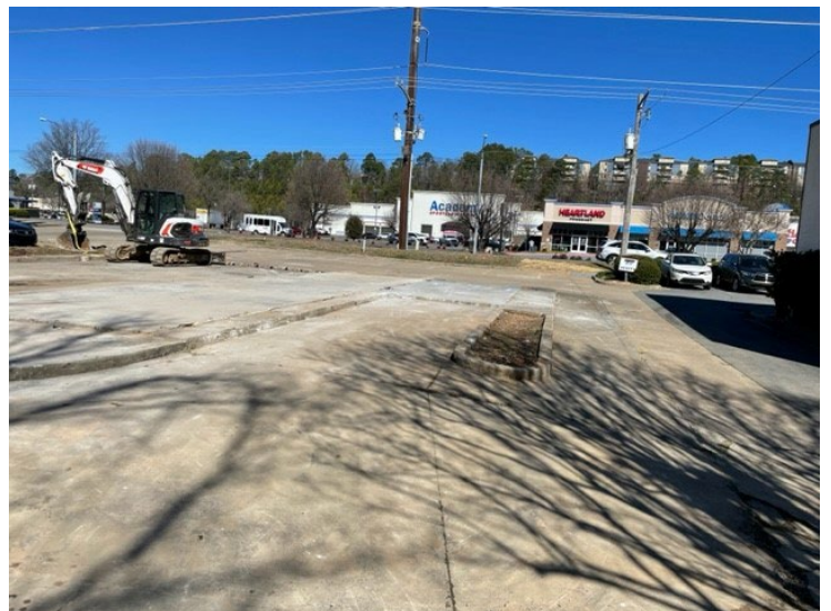
VIEW FROM SOUTH BOUNDARY TO MARKHAM (NORTHWEST)
