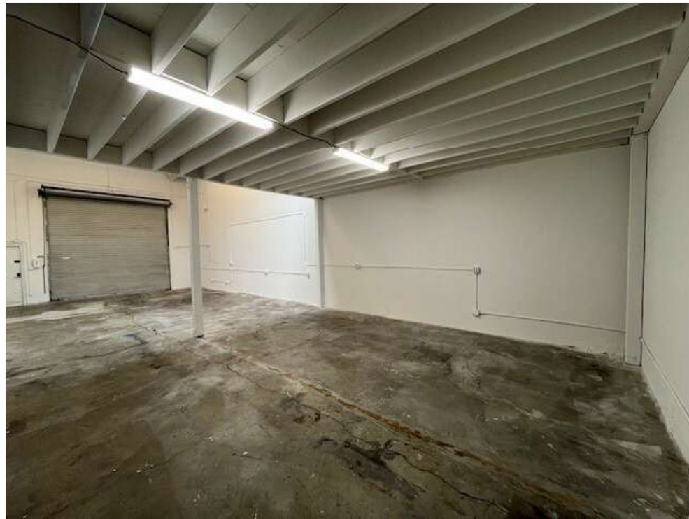
Lower Interior Industrial Space 2
