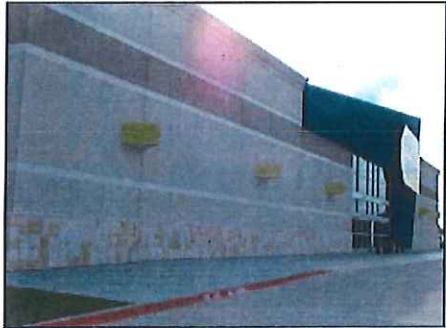
Figure 4: Building without Foundation Plantings
