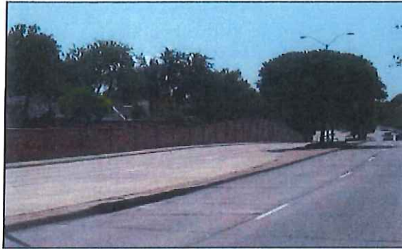
Figure 7: Screening Wall- Masonry
